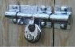
The bolt itself and the loops are case hardened, providing very high resistance to attacks from hacksaws or bolt cutters. The circular padlock has raised
