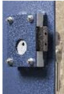
The door is locked by two 7-lever security locks.
